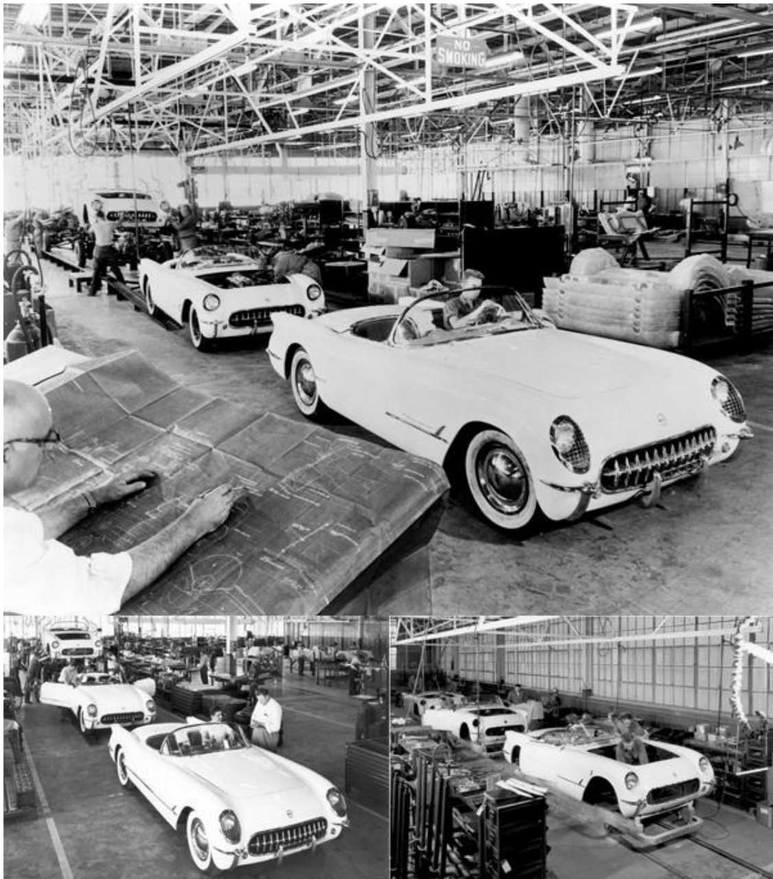
Inside the Flint, Michigan Plant
